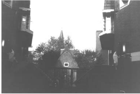
Figure 9.23 Hembrugstraat by de Klerk, use of space within the street block
